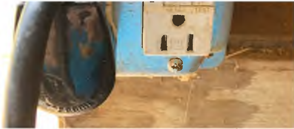
TOP: An enclosed fan offers ventilation with a reduced risk of motor or blades becoming damaged. MIDDLE: The left side and right side of the barn are wired separately at Wellmann's facility, which allows them to dedicate the left side for light switches and the right side for fans. BOTTOM: This box has switches with a reset button, which prevents the fuse box from blowing up should an appliance get too hot. Photos courtesy of Sharon Wellmann
